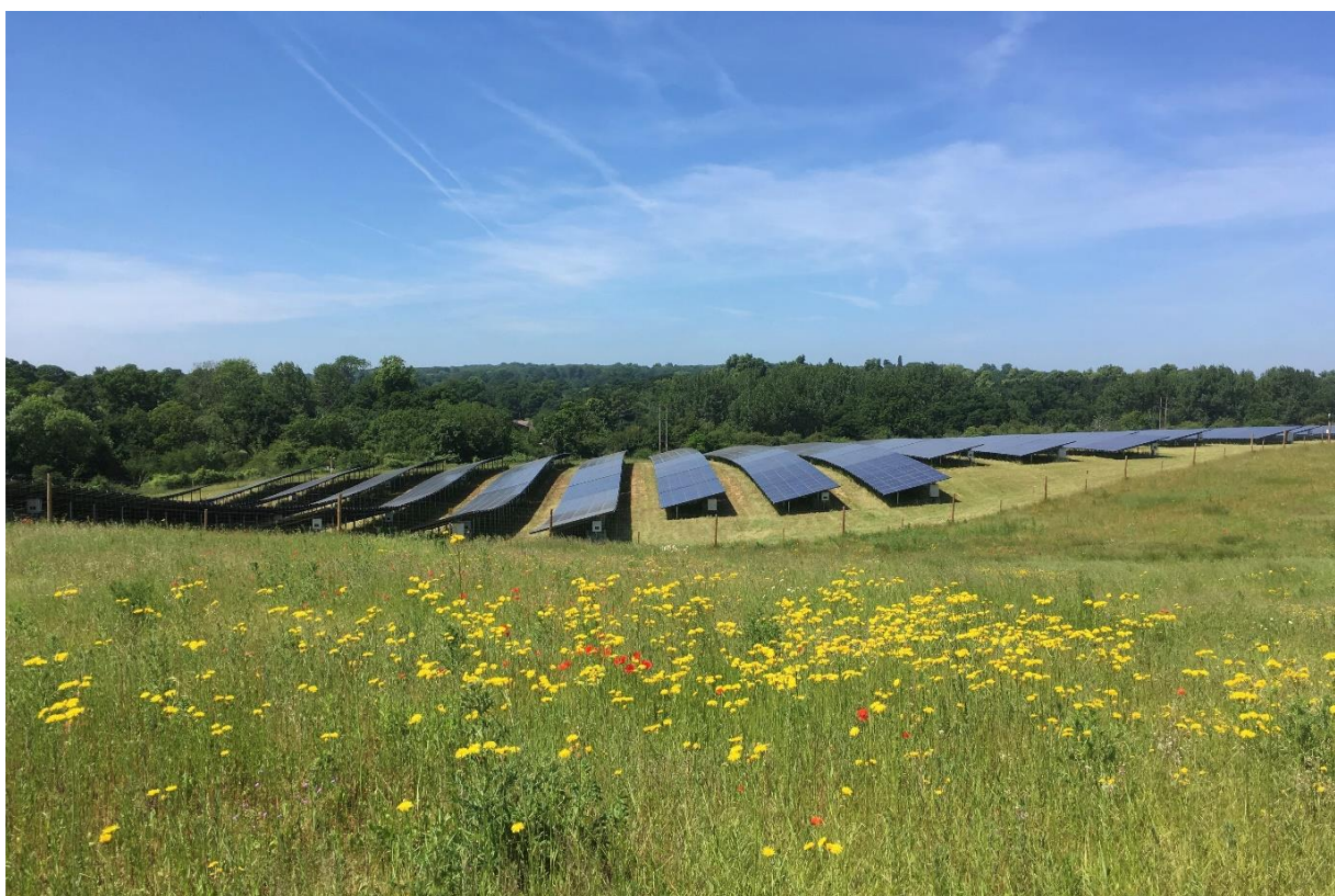
Southill Solar Farm
