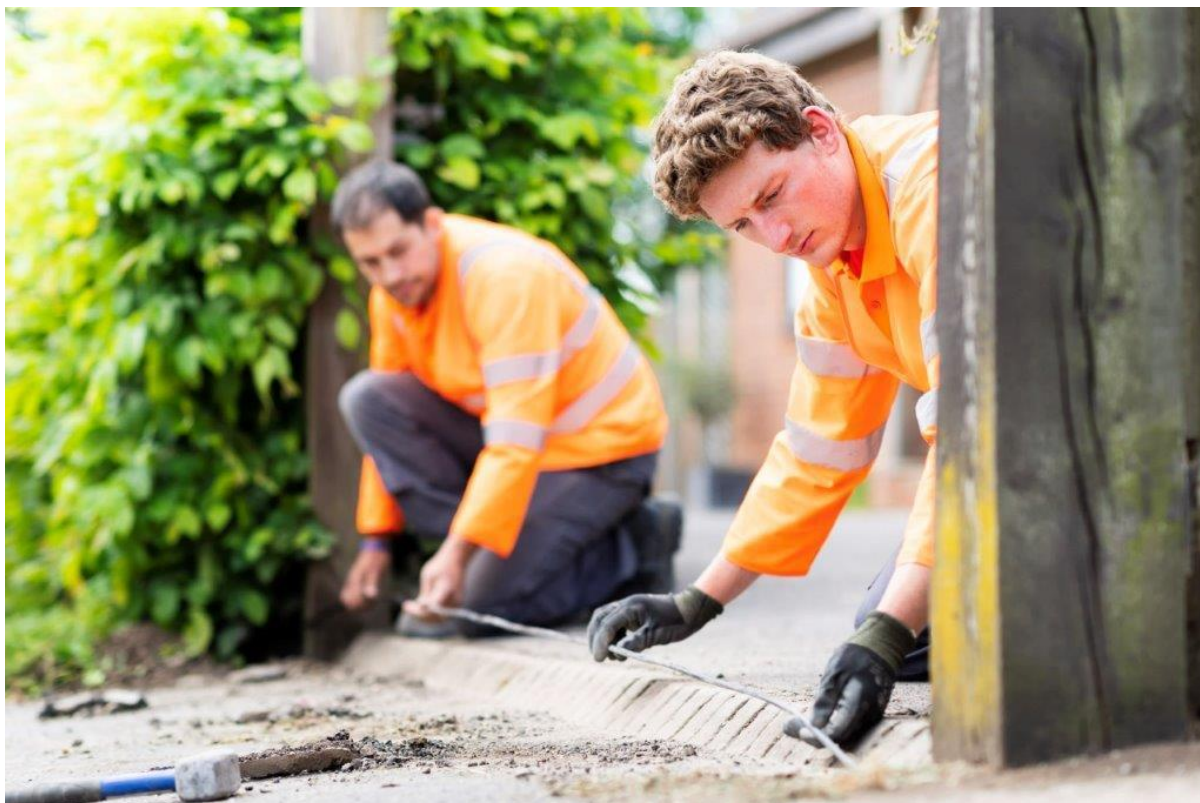
Gigaclear engineers laying broadband cable
